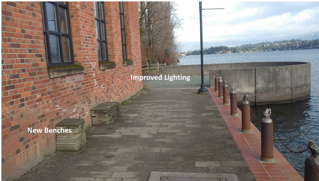
Diagram 3 Existing Plaza and East Side of Boiler Building with Approximate Locations of New Benches and Lighting (Looking North)
